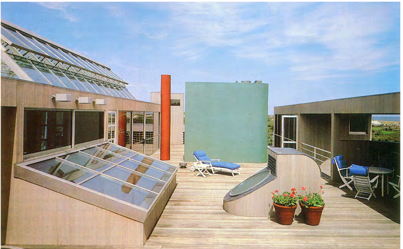
OPPOSITE: At the pool terrace, Mr. Gwathmey identifies the sequence of structural sections that correspond to the four internal zones of the house, left to right: entry greenhouse; circulation and living areas; and sunscreen. TOP LEFT: The entrance axis is encountered once again through a void on the south façade. TOP RIGHT: From the stair landing, an ocean view is framed by the sunscreen. ABOVE: The roof deck climaxes the structure's vertical organization.
