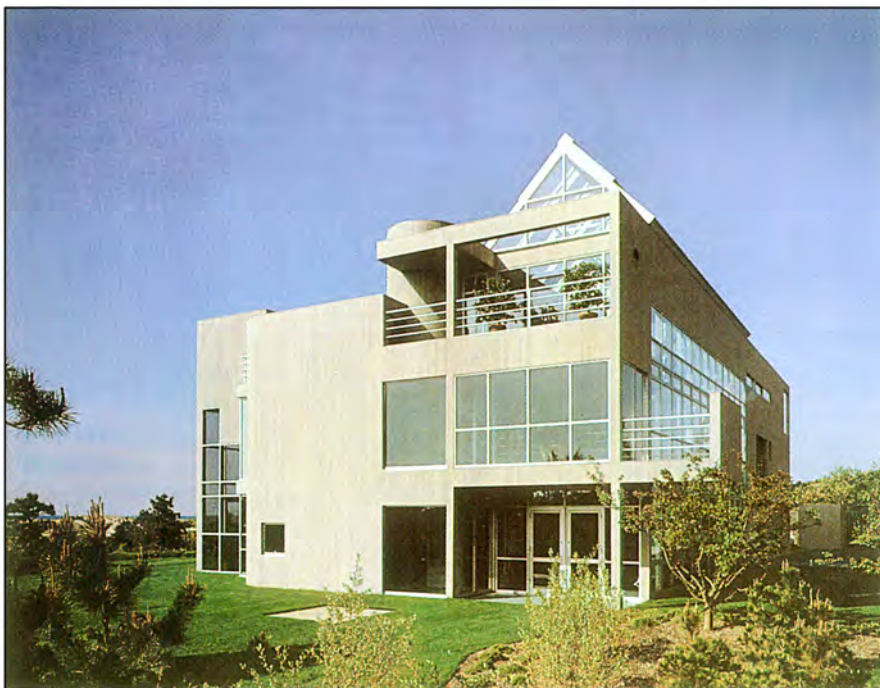
TOP: At the southwest corner of the house, the sunscreen becomes a significant formal element. ABOVE: The east façade displays a view of the gable-roofed greenhouse contained in the overall context of the house. OPPOSITE: A glimpse into the screened porch reveals examples of the Vienna Secessionist furniture assembled for the house—table and chairs by Josef Hoffmann.
